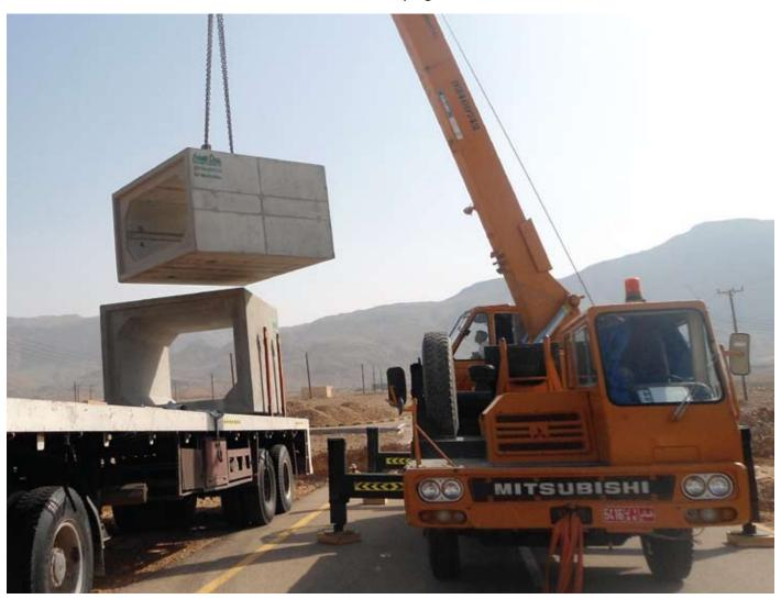
AMIANTIT OMAN CONCRETE PRODUCT BOX CULVERT GETTING INSTALLED IN CYCLE PHET DAMAGED AREAS
